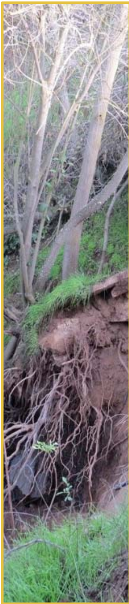
Seventh Street Storm Drain Repairs
